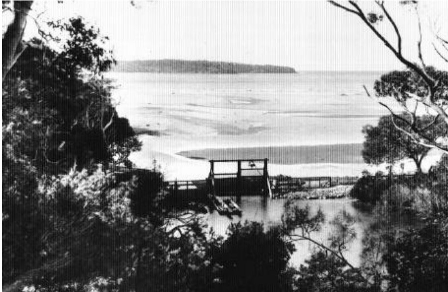
Figure 2-5: View over Simpson's Bay showing the stone walls and double gates of the fish hatchery (circa. 1910). Note the position of the entrance to Cabbage Tree Creek (and the lack of mangroves north of the gates).
