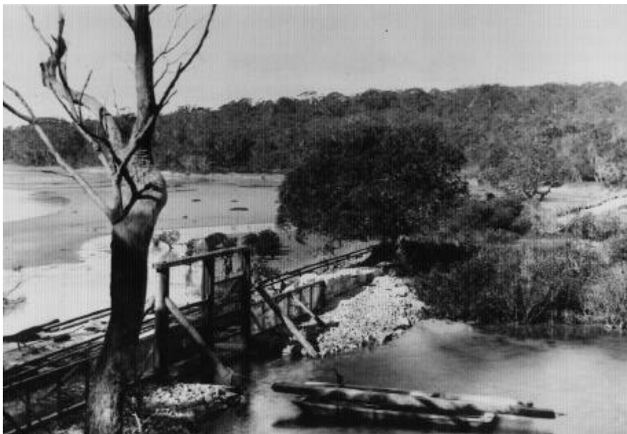
Figure 2-6: View to "Simpson's Hotel" showing the operating fish hatchery (circa 1910).
