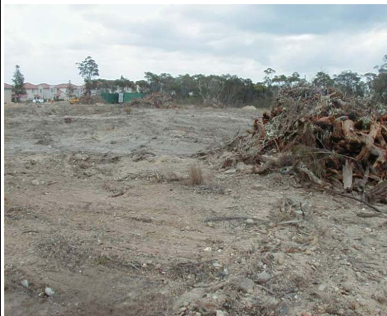
The site of the indoor sporting complex at Menai
